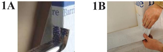
2. When using WindowWrap, make two cuts at the corner of the window opening so that the tape may be folded down the face of the outer wall. The open areas will be covered when the side pieces of WindowWrap are installed.
