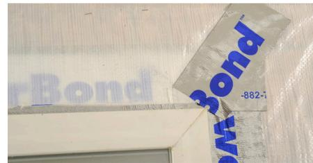
8. When installing arched topped windows follow steps 1B, 3 and step 4, then apply WindowWrap Flex around arch of window.
