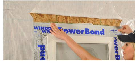
7. When done, fold the house wrap back in place over the header piece of WindowWrap and either tape, staple or use a piece of WindowWrap to secure.
