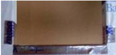
3. If using house wrap, the tape on the header section must be applied directly against the sheathing underneath the house wrap. Slit the house wrap at a 45 degree angle from the window corners and lift it up to expose the sheathing.
