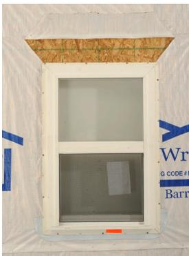
5. Adhere vertical sections of WindowWrap (5A and 5B) over the jamb (side) flanges and to the shear wall or house wrap. The vertical tape should overlap the tape at the bottom and extend 3" above rough opening at the top, preferably onto the exposed sheathing.
