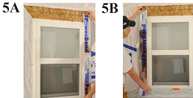
6. Adhere WindowWrap to the header flange and shear wall. Head section must extend beyond jamb sections on either side. Jamb (side) sections should not extend above head section.
