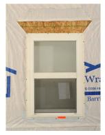
Adhere vertical sections of WindowWrap (5A and 5B) over the jamb (side) flanges and to the shear wall or house wrap. The vertical tape should overlap the tape at the bottom and extend 3" above rough opening at the top, preferably onto the exposed sheathing.
